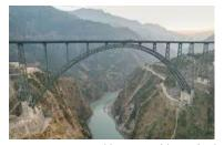
marvel is a crucial component of the Udhampur-Srinagar-Baramulla Rail Link (USBRL) project, which aims to connect the Kashmir Valley with the rest of India by rail. Constructed at a cost of 1,486 crore, the bridge spans 1,315 meters and is designed to withstand extreme conditions, including earthquakes and high wind speeds .
